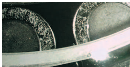
Roller end wear caused by over tightening, lubrication degradation, or lack of lubricant.
