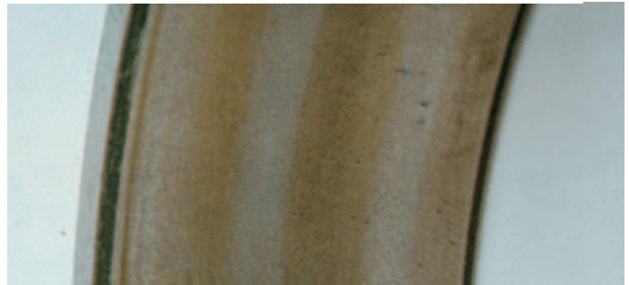
Pitting of the race, as a result of debris in the lube causing surface deformation.
