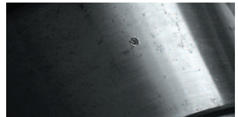
Surface appearance caused by electrical arcing during welding.
