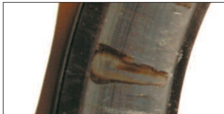
Cup shows considerable corrosion. This will develop in spalling.
